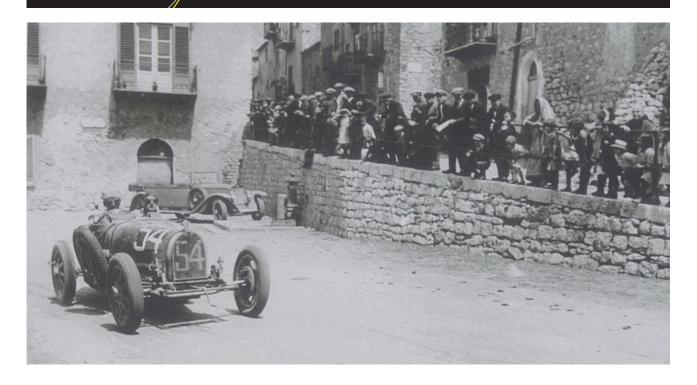
On the 6th of May 1928 Heusser raced 4814 in the Targa Florio. Car No. 54 it sadly retired on the 4th of 5 laps. From the picture above we can see the radiator is the 350mm size, there are no extra louvers on the bonnet but the blower hole is visible. The car is also darker as it is believed that Heusser painted it red.
